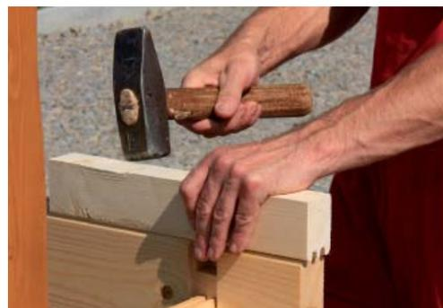
Assemble the remaining plank rows as described above. At the door, simply slide the planks in the door frame.
