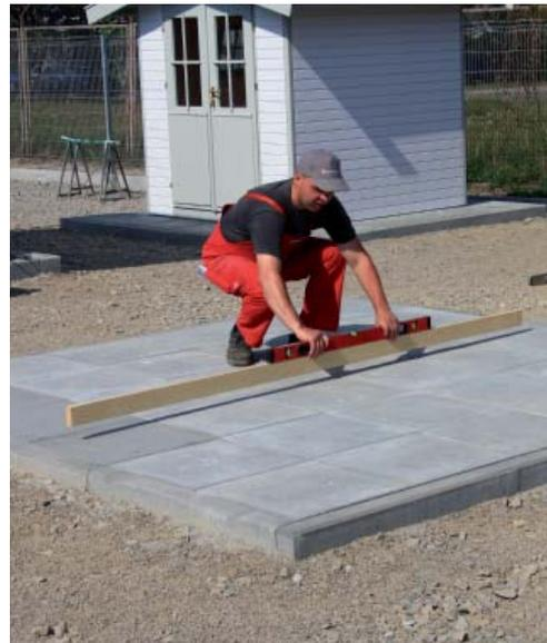
As a basic principle, only build your summer house on a level surface. Check your foundation prior to assembly!
