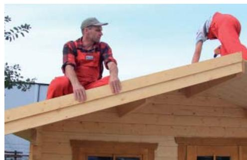
Now mount the **gable boards** at the front and back. Fix the gable boards with screws to the roof boarding and the ridge/centre purlin; the spacing between the upper edge of the gable board and the upper edge of the roof boarding should be approx. 5-6 cm.
