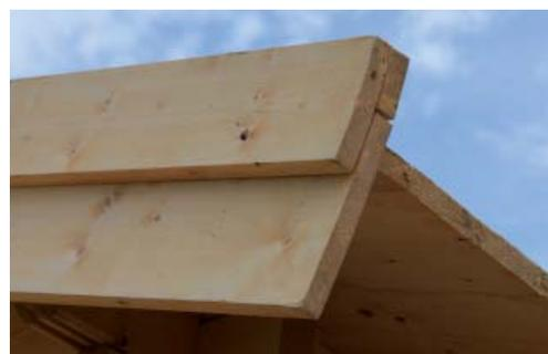
Mount the **fascia boards** with screws to the roof boarding.
