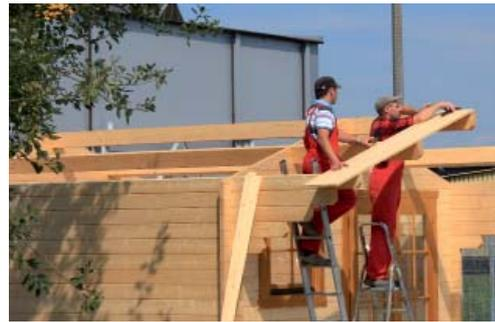
Now nail the boards twice to the ridge/centre purlin and the fascia board. Lay the roof boarding all the way to the back. Measure in regular intervals to ensure that they are properly aligned and that the spacing to the wall is consistent. The backmost (final) board needs to be cut to size in most cases.
