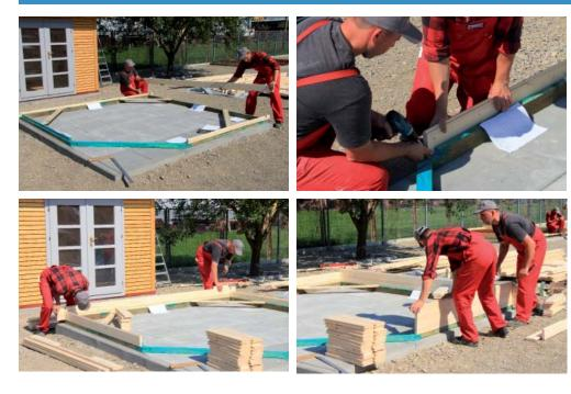
Lay the pictures contained in the drawing at the respective wall sides to us as a reference so you can always check to make sure all plank rows (and windows) are properly placed.
