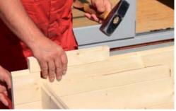
in this fashion. To avoid damages to the planks use the provided block of wood to connect the planks firmly. Repeat this step until you have inserted the planks with the window opening. Now mount four more plank rows in the rear part of the summer house to insert the window later on.
