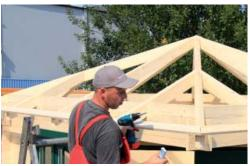
nected with each other. Screw all rafters together and to the wall elements. The roof boarding is already pre-cut for all roof sides and marked with numbers/letters. You can also find them in the drawing.
