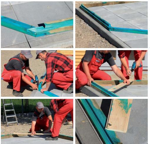
Lay out the base frame on your foundation as shown in the drawing. Lay it out so that the door is located at the desired position. Screw the frame together beginning at the corner opposite the door. Make sure the corner is at a right angle. To keep the corner from moving, screw a board (leftover pieces from the package) opposite the corner on the upper edge of the frame.
