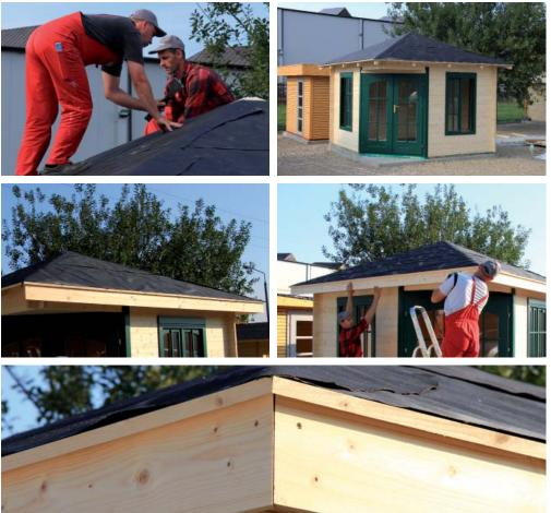
Now lay the next sheet of roof felt above this sheet. Also allow an excess on the left and right-hand side so that now there is approx. 30 cm of overlap over the lower sheet. Attach the felt. Repeat this step in this fashion for the remaining roof areas.
