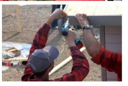
The roof boarding is already cut to the correct length so that you only have to lay the boards from front to back.
