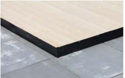
If you also want to protect the floor with roofing felt, pull up the excess material and fix it to the fascia boards of the floor with small nails or staples. Cut off any remaining excess material with a cutter.
