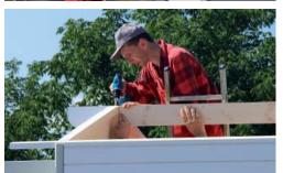
Now screw the fascia rails and the ridge purlin to the respective components with the proper tension.
