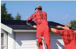
Lay the sheets so that the next layers always overlap the underlying sheet at the upper edge by approx. 20-30 cm.
