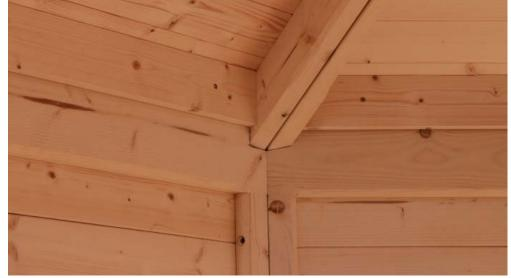
Now take a screw clamp and tighten the adjusted roof element at the roof overhang (outside) and screw them together from the left and right hand-side. Place two small pieces of wood underneath the clamp to protect the wood.
