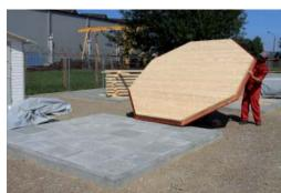
Now take screw clamps and fix the floor elements where they meet and screw them together with the provided screws (approx. 6-8 screws depending on the model).
