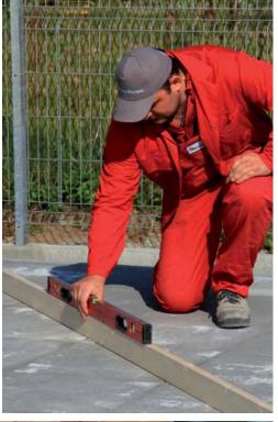
As a basic principle, only build your summer house on a level surface. Check your foundation prior to assembly!
